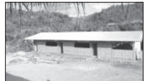
The bamboo school - three classrooms with a concrete floor and block room dividers and end walls. In the middle of the project, the contractor demanded four times the pay he was receiving. Cat couldn't pay him, and he left. When four Australians wrote they were coming to visit, Cat didn't want to be bothered because of her deep concern over the school. She went to pick them up anyway in Bangkok. One of the men said he didn't know why he had come. He wasn't an Adventist or even a Christian. He wondered what a retired contractor could do for a mission. Cat was ecstatic. She said, "You can build the school." And he did! He trained the students to lay blocks and together they built the new facility, with funds donated by members of the Carolina Conference.
